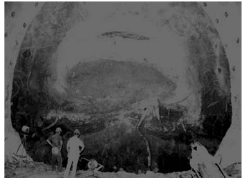
Fig. 7: Old collapsed tunnel during re-excavation.
