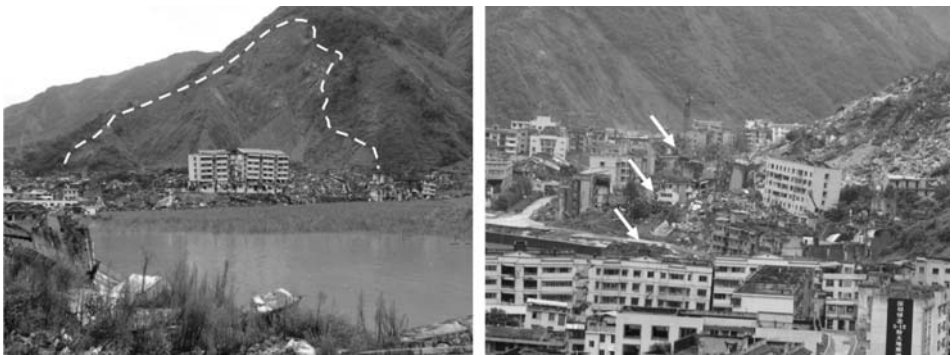
Fig. 7: Views of Beinchuan town which was almost totally destroyed ( ESI_{2007} = XI, XII ) due to the combined action of the seismic fault Yingxiu-Beinchuan (arrows) and the huge landslides.
