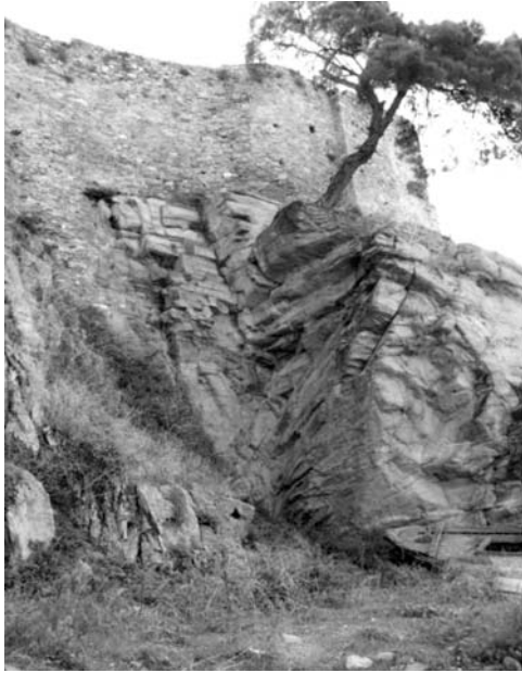
Fig. 2: Location P1. A fault intersects the slope forming a huge rock wedge and a wide fractured zone. The Wall fills the gap between the two sections of the fault.
