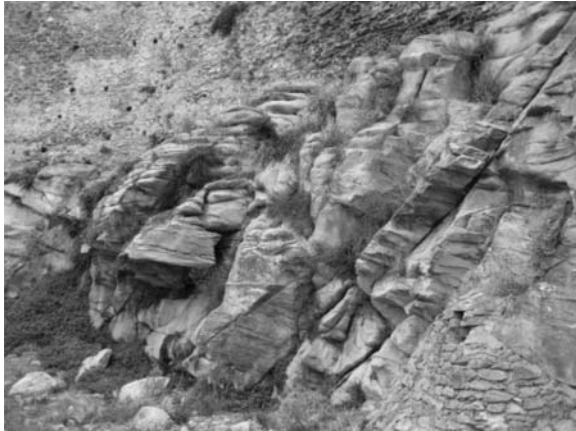
Fig. 6: Part P6. Several rock wedges are formed, to prevent them from sliding the underexcavated rock blocks were sub founded by the use of masonry walls – fills (lower right corner of the picture).
