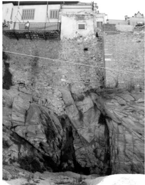
Fig. 3: Location P4. An intensively fractured zone caused by a fault. The wave erosion caused intensive underexcavation to the slope.
